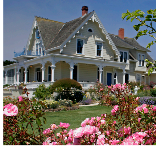
PHOTO: RITA CRANE STUDIO
